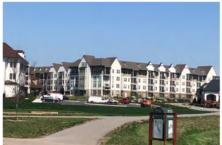
Apartment Building | Prairie Village, KS
