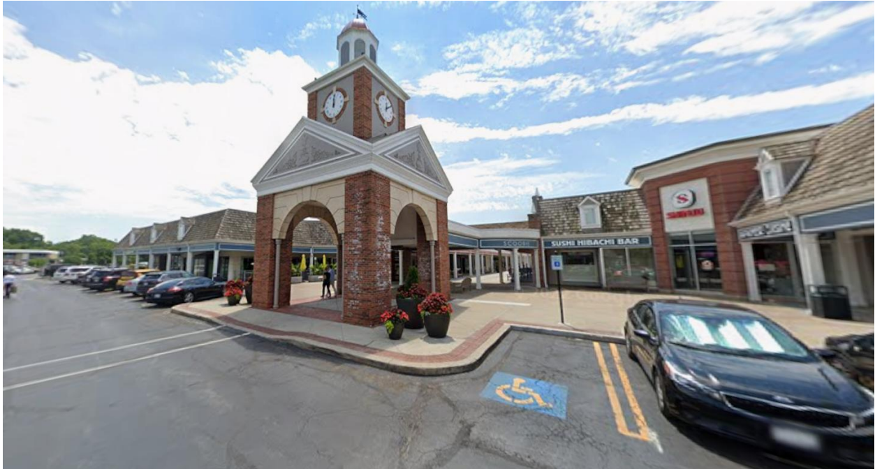
Looking southeast at the north entrance to the interior courtyard
