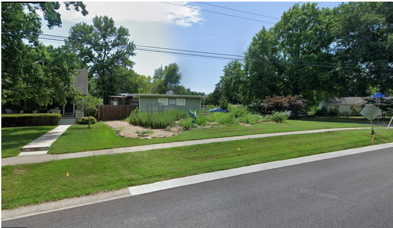
Looking southeast at the intersection of W. 79 th and Reeds Road - fence on left
