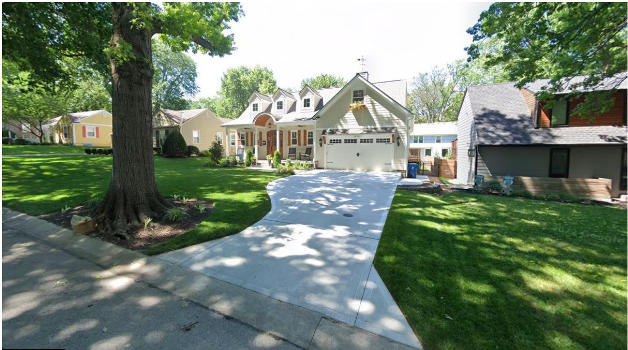
Looking southeast from W. 73rd Street – proposed patio expansion in rear yard.
