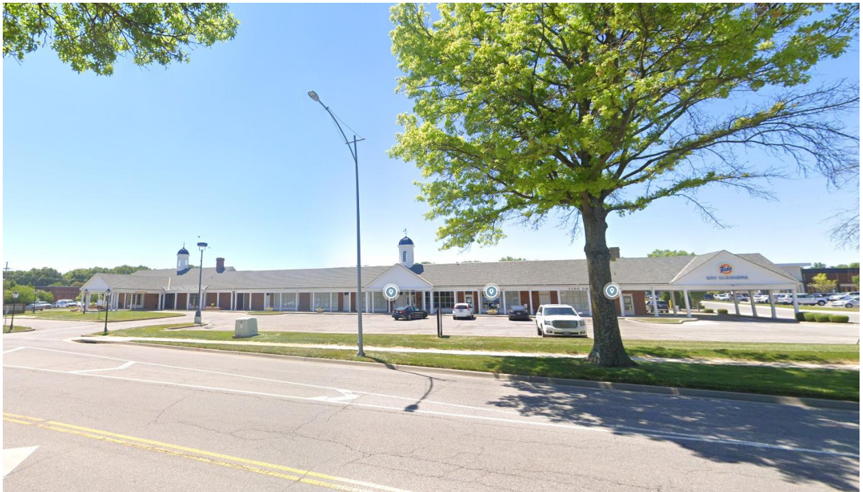
Looking southeast on 83 rd Street
