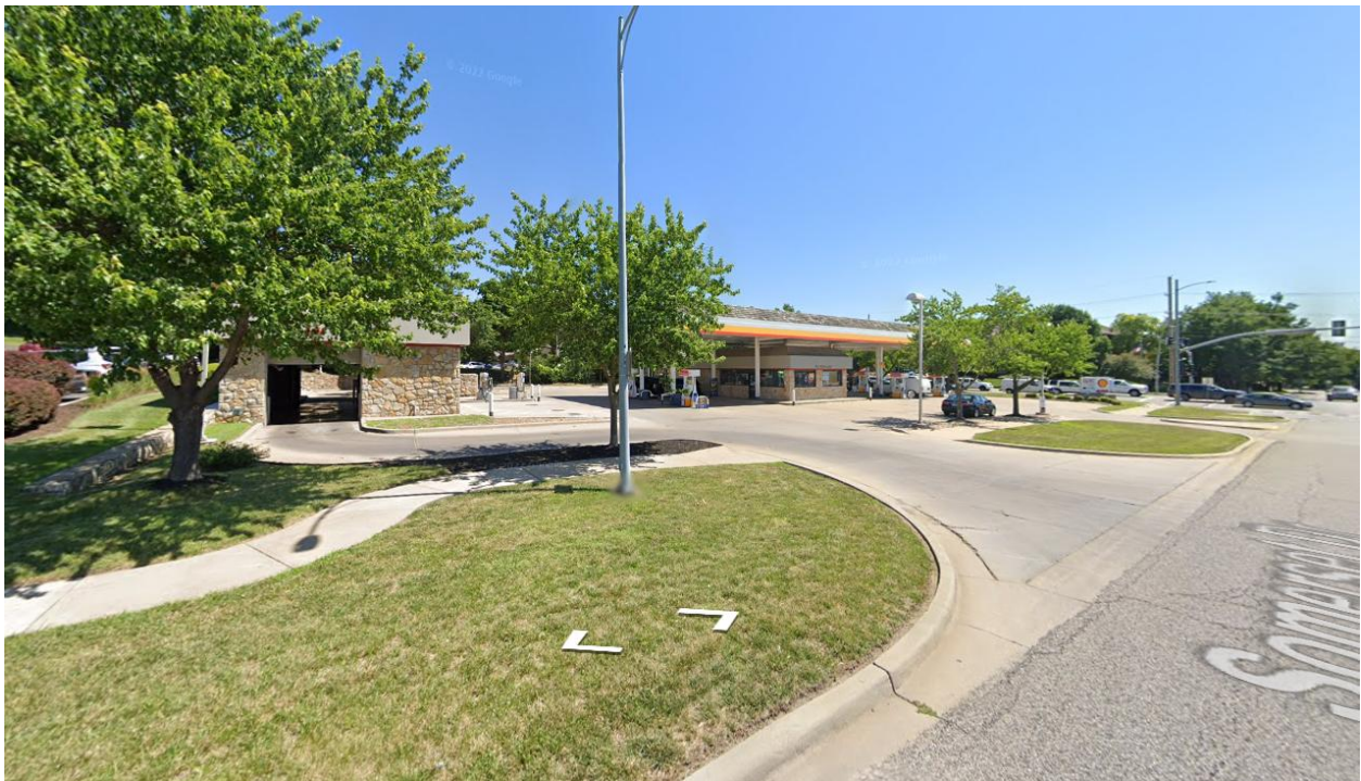
Looking east on Somerset Drive
