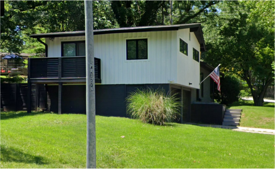
CURRENT SIDE PROFILE OF BLOCK FROM STREET PAINTED A DIFFERENT TONE. ALL NEIGHBORS WITH SIDE SPLITS HAVE THIS BLOCK EXPOSED
