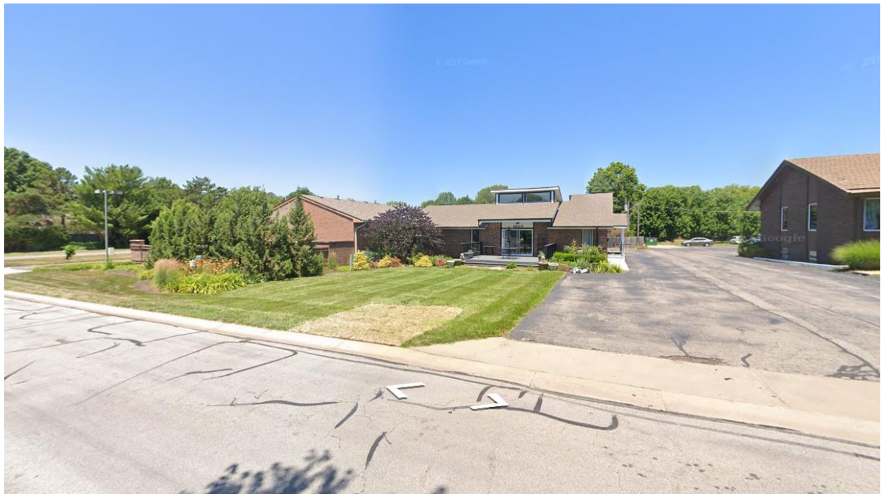
Street view looking north on W. 89 th Street
