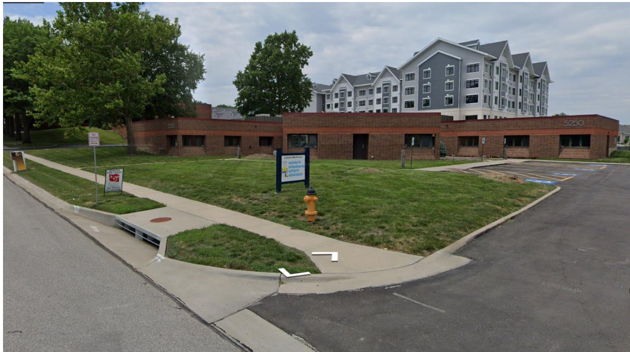
Street view looking northwest on W. 94 th Terrace – sign will replace existing sign.
