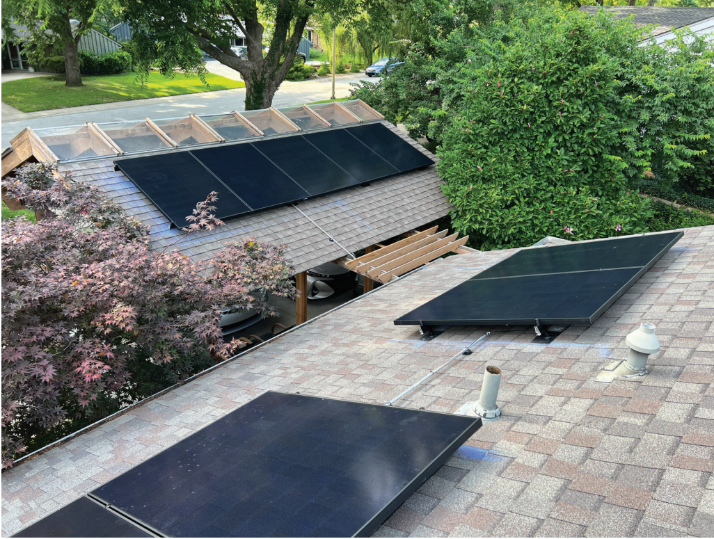
ROOF VIEW FACING WEST, CARPORT EAST FACING
