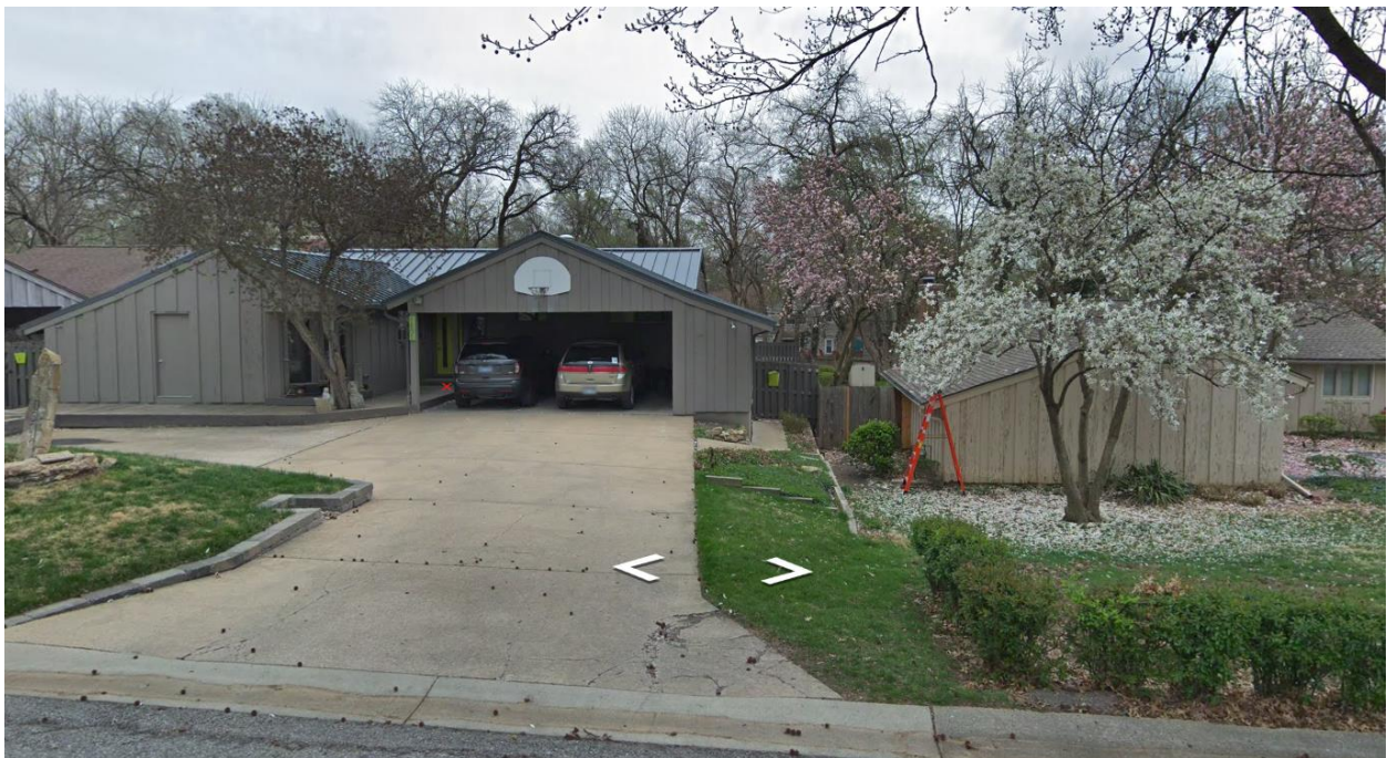
Subject property with existing retaining wall on right.
