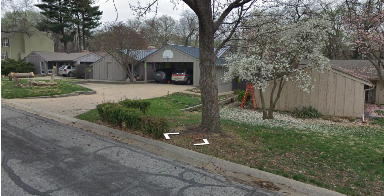
Lot and property on left, existing retaining wall in foreground.
