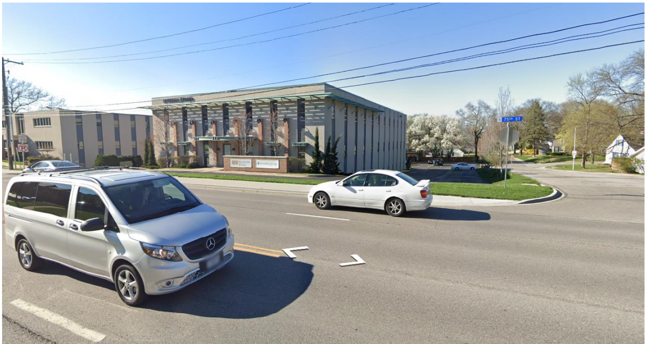
Street view looking north on W. 75 th Street
