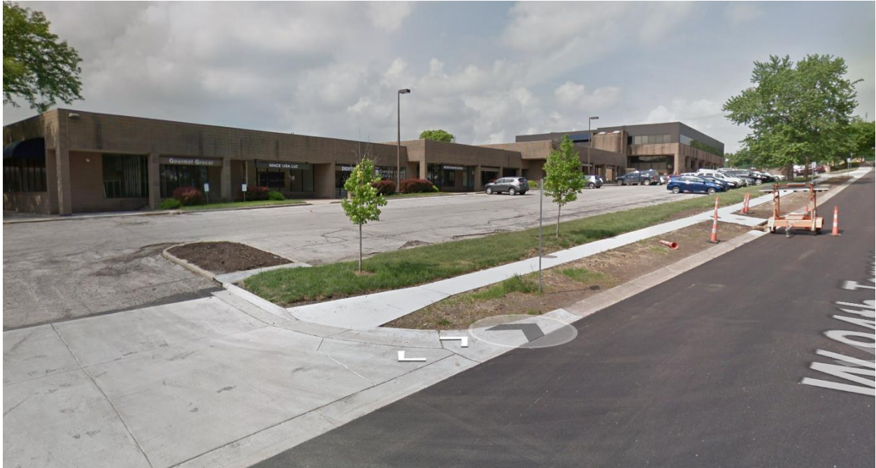
Street view looking southwest at from W. 94 th Terrace.
