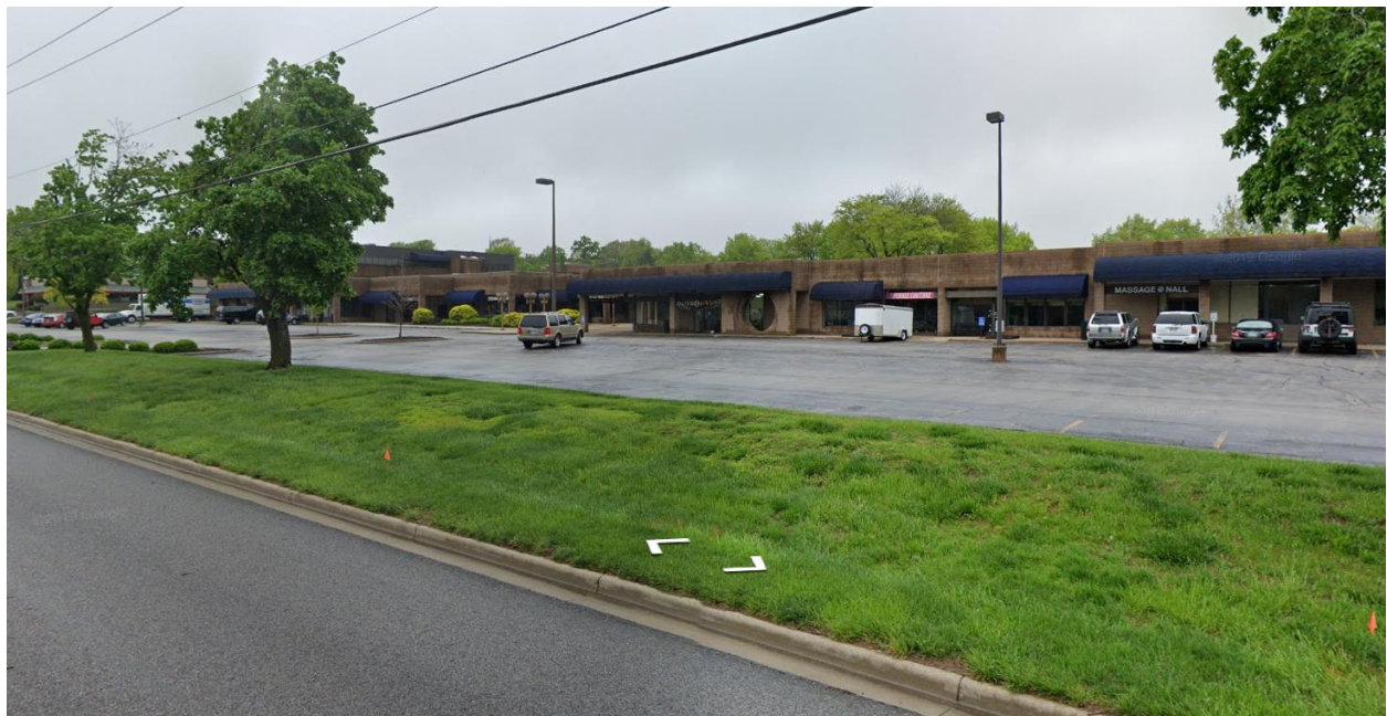
Street view looking northwest at the building frontage from W. 95 th Street
