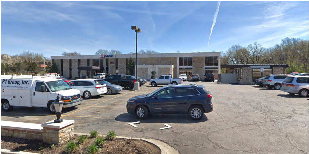
Street view looking east at the rear of the building (internal street).
