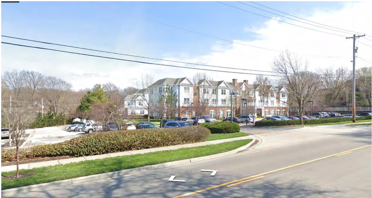
Street view looking east from Mission Road
