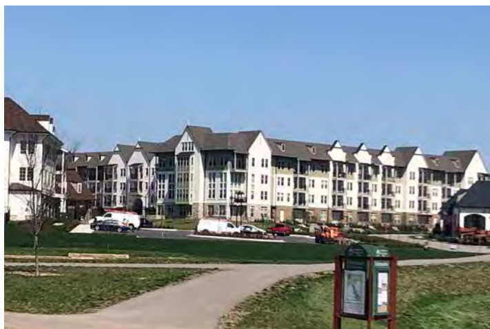
Apartment Building | Prairie Village, KS
