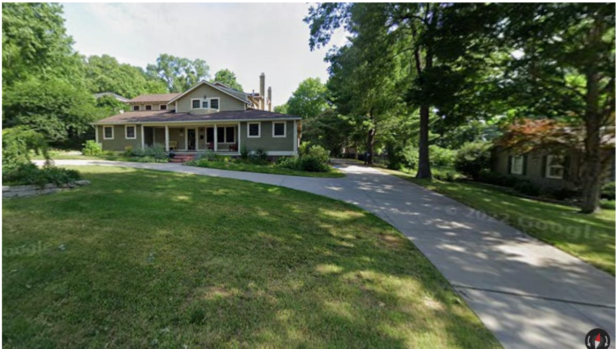
Looking north at 5112 W. 67 th Street - accessory building location in background to the right.
