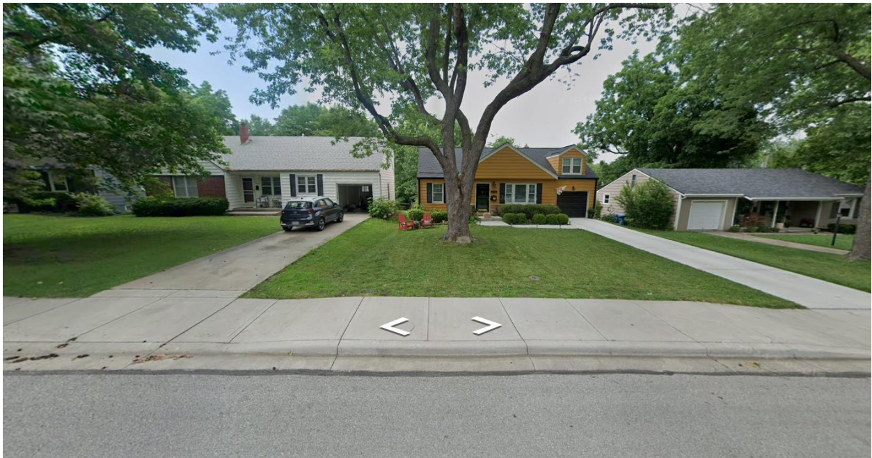
Looking north from West 72 nd Stret – Subject in the middle; subject lot line on left.
