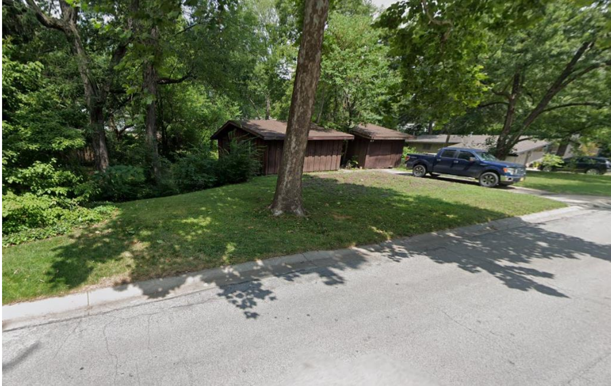
Looking northeast on West 71 st Terrace
